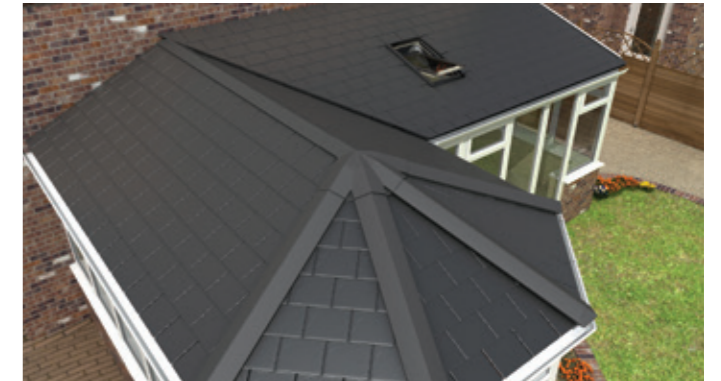
Chosen tile is added ensuring weathertightness and the gutter and external trim are secured in place.
