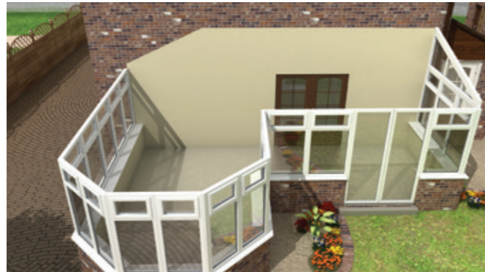
The vital first step is to remove the entire existing roof.
